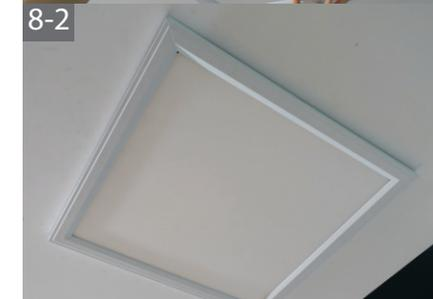
**Step 8:** Push the luminaire on to the ceiling. Make sure the 4 hooks are inside the luminaire and slide the luminaire forward until you hear a clicking sound.
