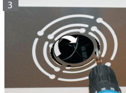
**Step 3:** Align the holes on the surface mounted kit with the holes on the J-Box. Tighten 2 #8-32 screws, rotate the plate to your desired position and fasten the KA3.5x20mm screws into the ceiling until the kit is flush with the ceiling.
