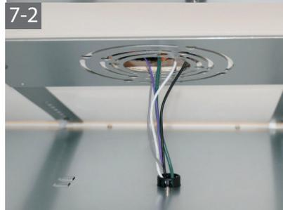
**Step 7:** Place the wires into the J-Box.
