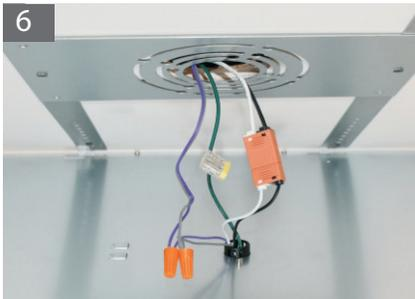
**Step 6:** Plug the female connector of the luminaire into the male connector of the AC input wire. The ground connects to green wire. Dimming wires connect according to the same wire color.
