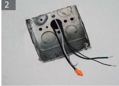
**Step 2:** Turn off power. Insert the L, N wires of the J-Box into the male connector.
